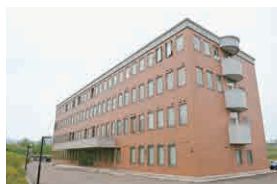
看護棟 (6号館) Nursing Dept (Bldg 6)
